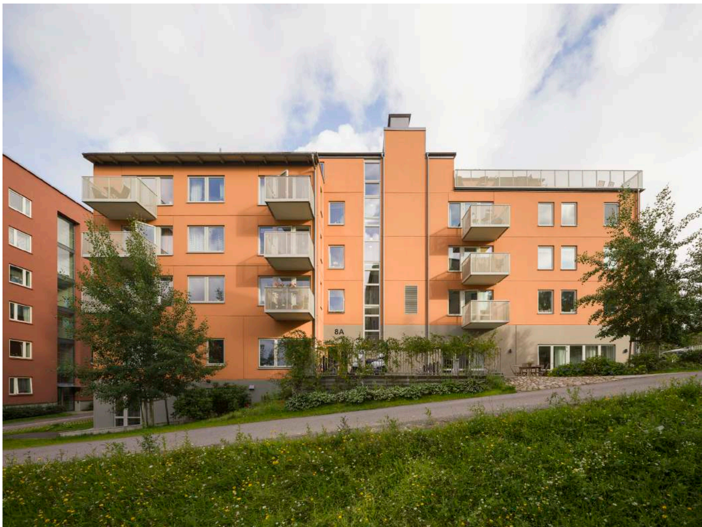
The facade towards northwest.
